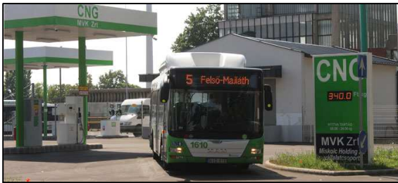
Figure 10 CNG fuelling station in Miskolc, Source: http://mvkzrt.hu/mvk-cng-toalloallas
